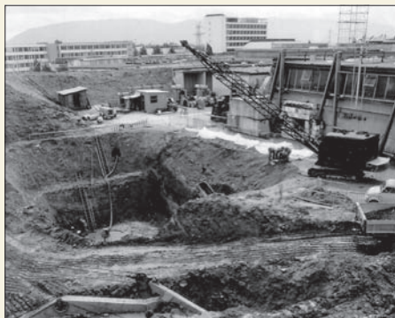
Excavation of the hole for the underground laboratory of the ISOLDE project. The project will use extracted proton beams from the 600 MeV synchrocyclotron in the adjacent building (right).
